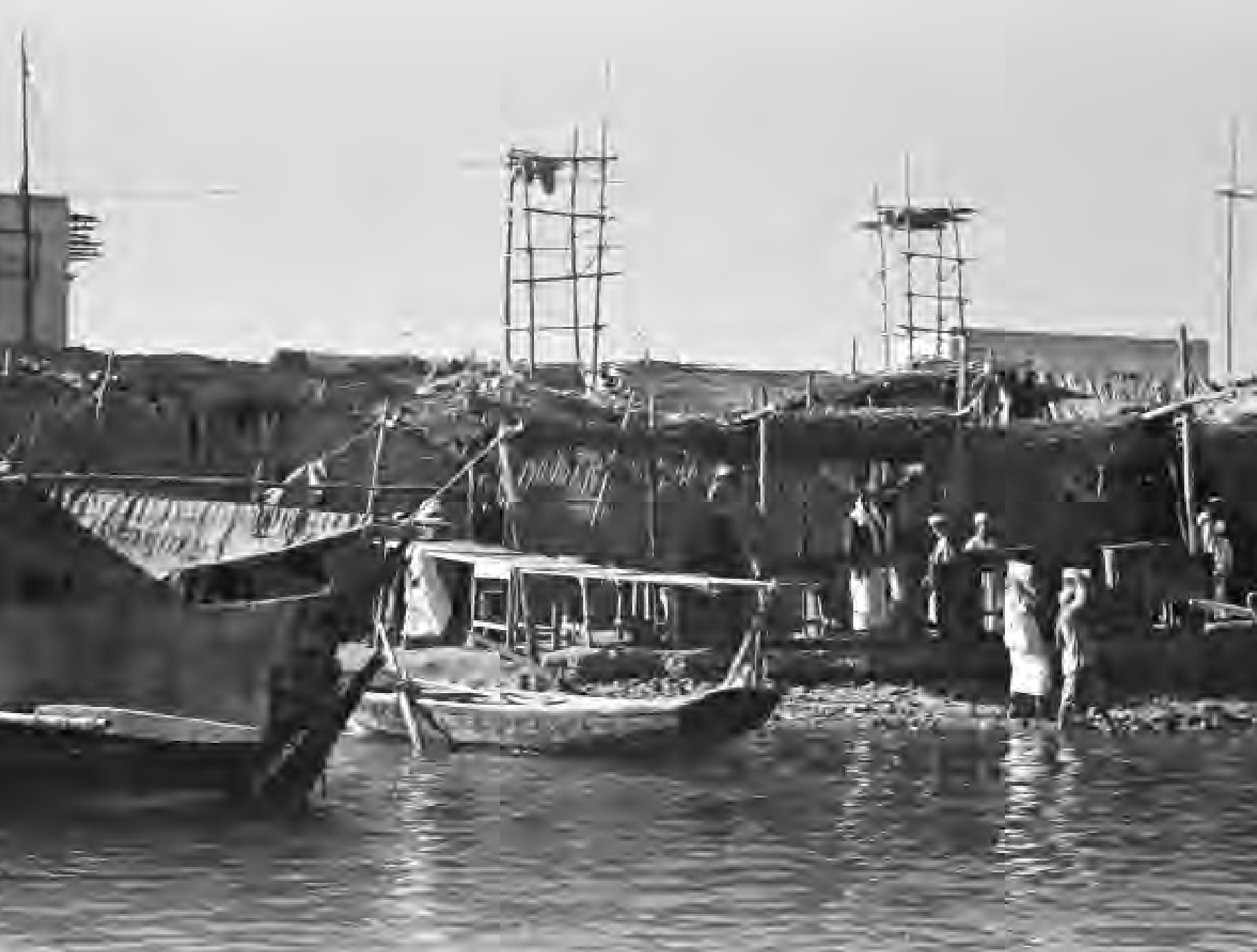
Dubai, May 1949. Framework for wind towers constructed annually before the summer
