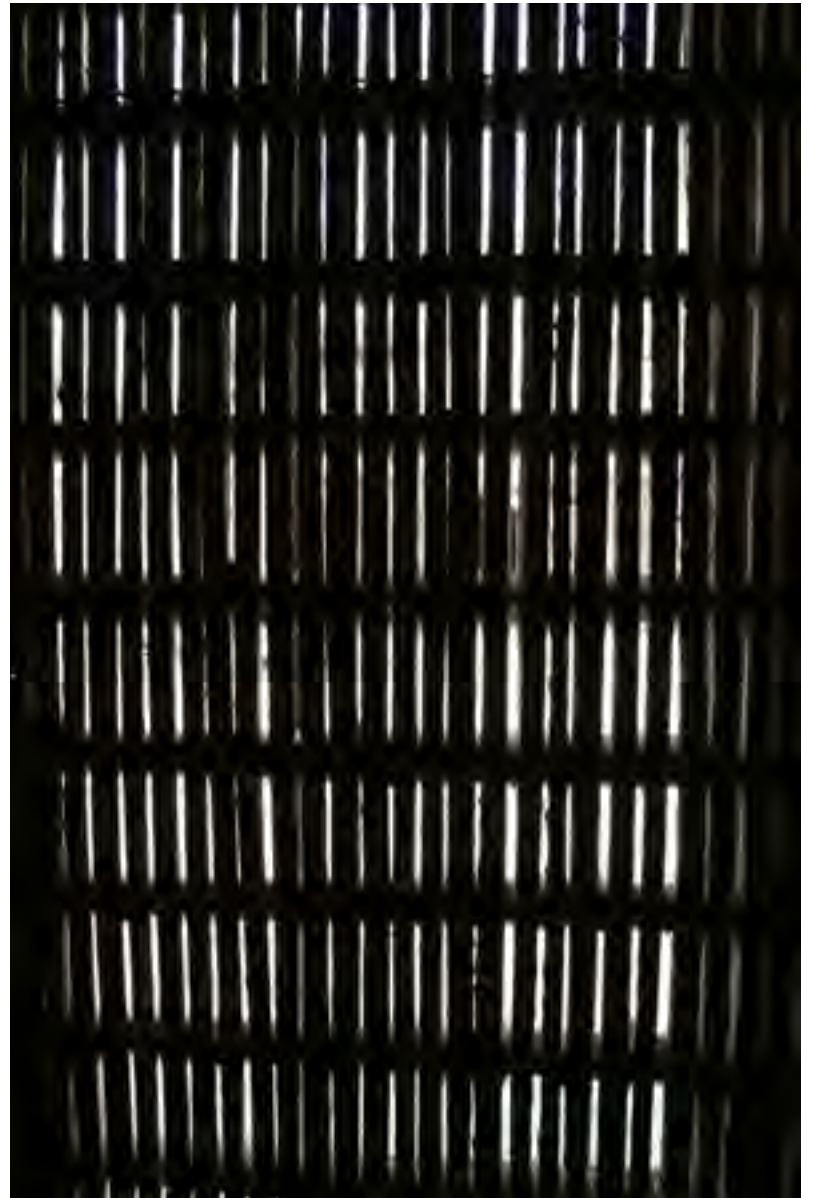
Details of Arish in Ajman. Typical slot (50 cm gap) for air intake covered traditionally with sailing canvas
