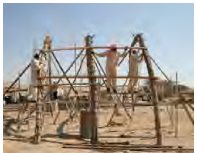
Series of tests aimed at creating a full-scale mock-up and evaluating structural capacities of palm leaves, July–November 2009. Tests were carried out by the author at ADACH's Sanaiya workshop in Al Ain with the assistance of ADACH conservation staff
